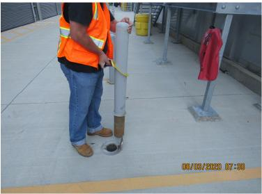
With the bend in the handle facing down, slide Bollard Lifter down over the top of the bollard.
